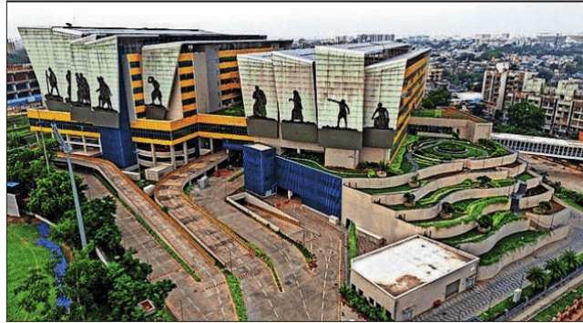
Designed as a twin structure, the hub earmarks space for offices, commercial development, and retail
